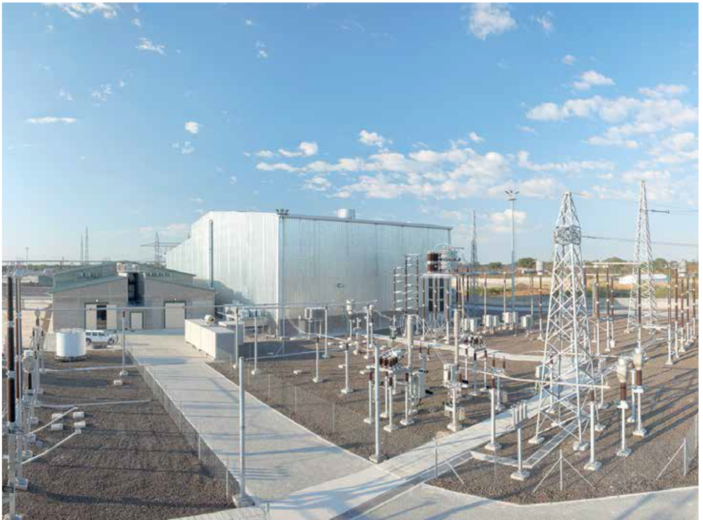
HVDC Light® station.
